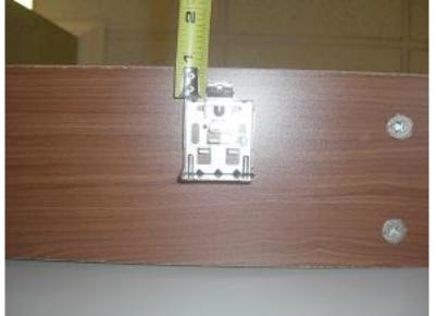
With mounting screw already in magnetic driver, attach bracket to sill Use two screws for each bracket Repeat for second bracket on opposite side If cell shade width is over 47" use third bracket provided for center of shade
