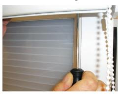
To remove the blind, push the lip of the bracket at the back of the cassette upwards using the head of a screwdriver. This will free the back of the cassette. Carefully remove to avoid damage to the blind.
